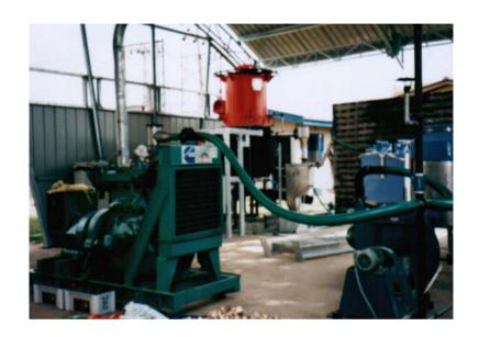
Energy Forum is in the process of installing a 40kW pilot dendro power plant in Wadakahakiwla village in Moneragala District, the first ever in Sri Lanka in an offgrid community setting. The community operated power plant provides 250W of environmentally healthy electricity to 100 households, while the necessary technical and institutional infrastructure to operate. maintain, and monitor and evaluate it are provided by the Energy Forum.
